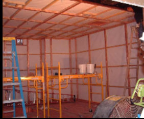
RF Shield Near Completion
